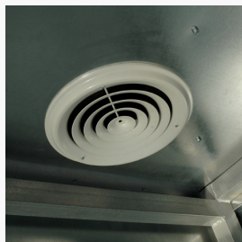
Extraction et aspiration VMC
